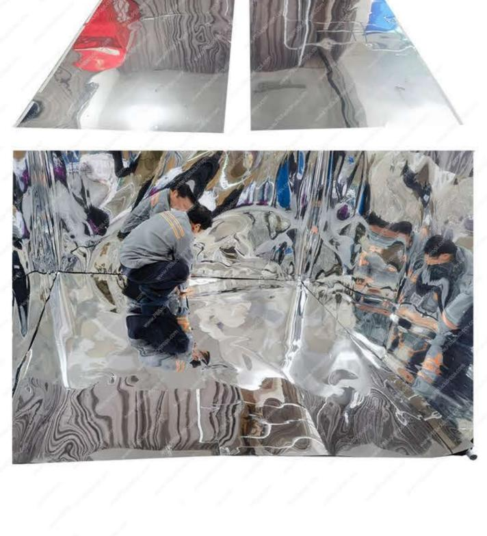
3. The entire arch is secured by a reflective film with hook velcro on its back
